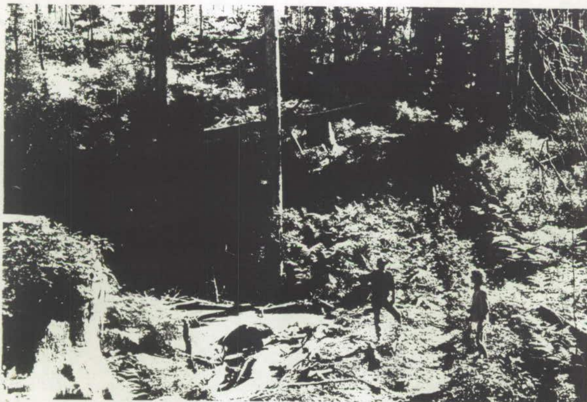
Plate 7.11. Earth crossing in C200 site 3. Filter strips have been cleared and sediment transport into drainage lines has resulted.
